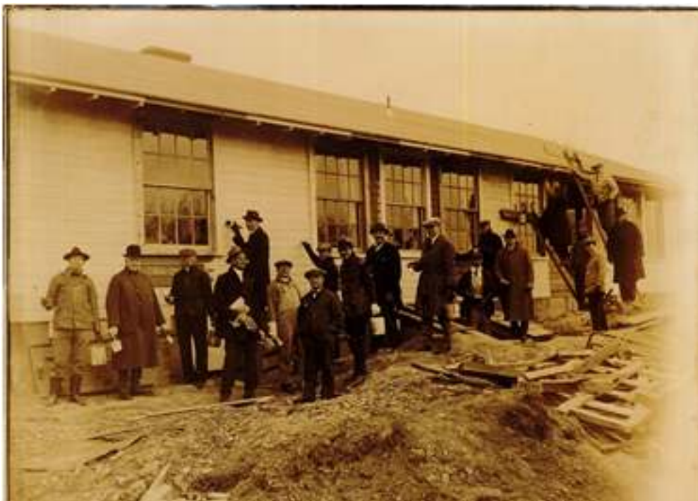
Painting the outside walls during construction of the Canandaigua Rotary Preventorium
